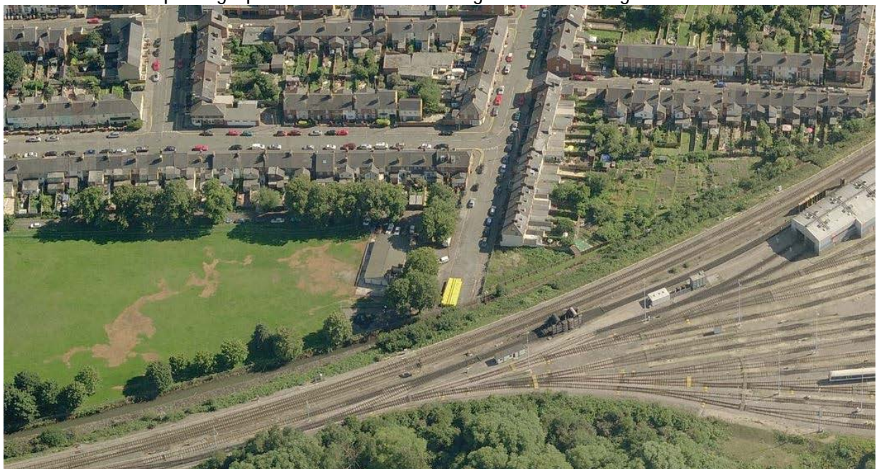
Aerial view looking south (prior to demolition of Fairview Community Centre)
